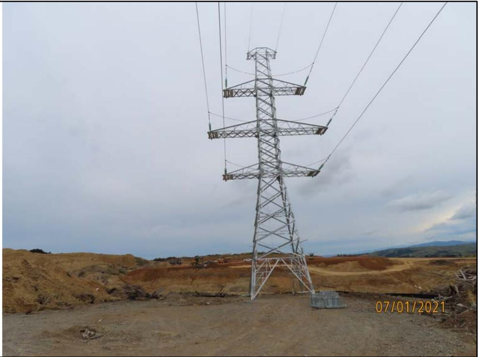
This picture shows Tower 38 where two circuits are bonded together. If and when Mercury's Puketoi wind farm is connected to the Plantation substation the circuits will be returned to individual independent circuits.
